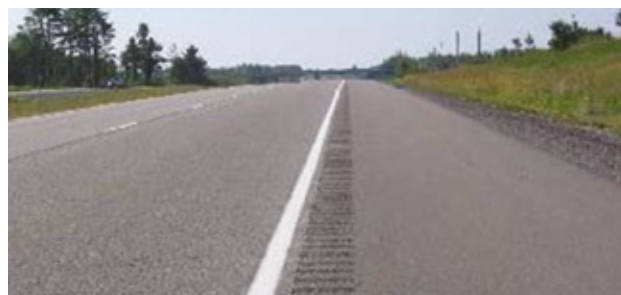
Illustration 60: Research in the USA showed that continuous hard shoulder rumble strips, also used along motorways in the UK and Canada, can reduce single-vehicle run-off road accidents by approximately 20% (Griffith, 1999).
