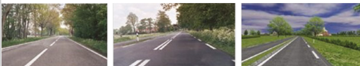
Illustration 55: Example of a distributor road in different road layouts: traditional, ERC and according to a real safe system approach
